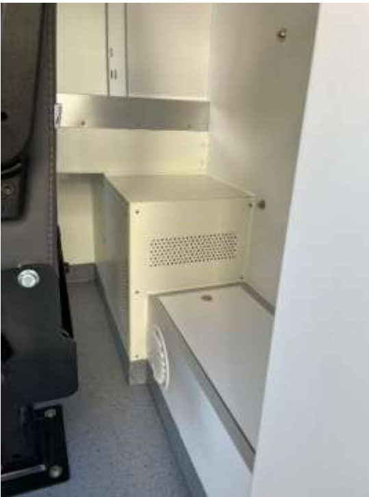
7 Negative Pressure & sec. battery Boxes
